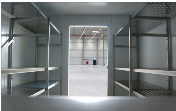
Interior walls and ceiling: stainless steel Heavy duty shelves. Shelf height: 1.800 mm 4 shelf levels standard. Additional shelves optional. Room lighting with motion detector standard. Robust stainless steel trolley ramp for safe and convenient access.
